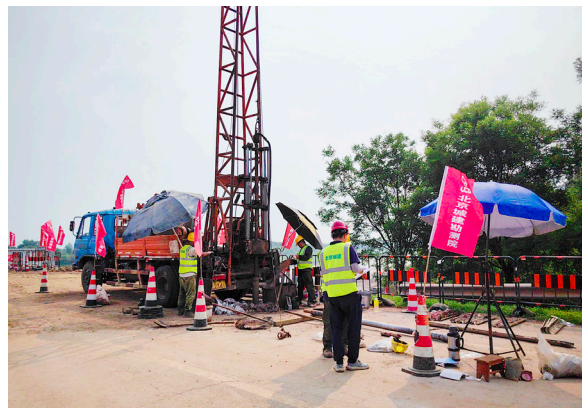
Work site of the emergency rescue team in Pinggu District
