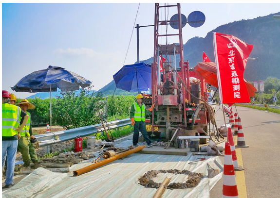
Work site of the emergency rescue team in Miyun District
