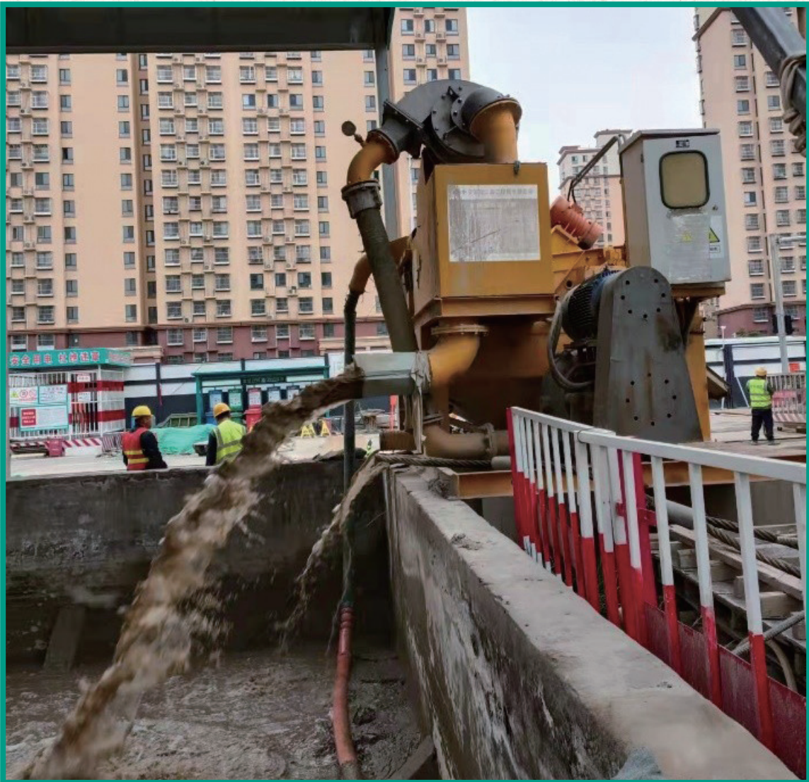
Picture: Process of slurry separator separating the slurry
