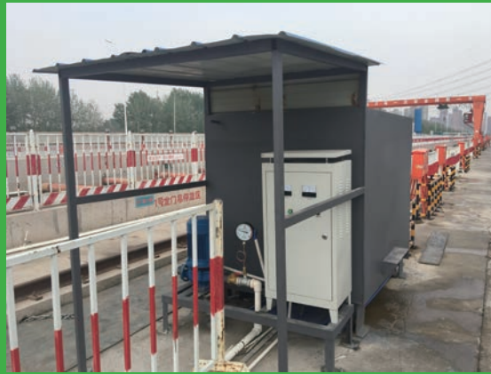
Picture: Variable frequency booster pump on construction site
